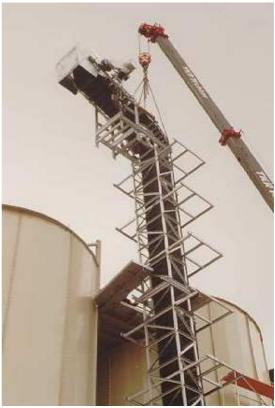
Elevator to extract from a pit for Metro construction
