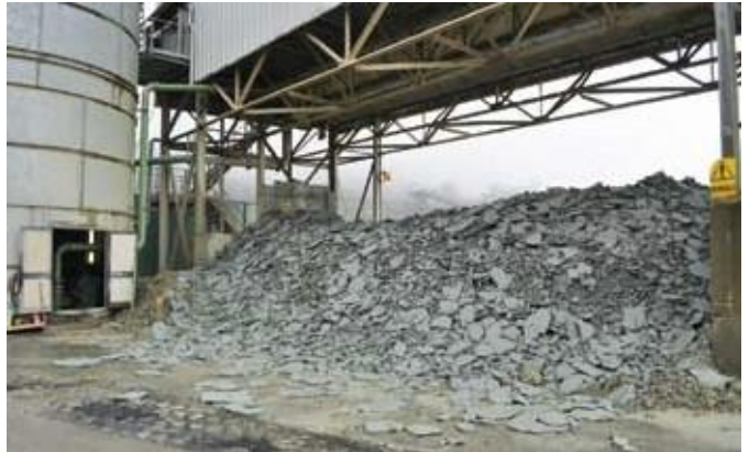
Concentrated slurries by PEMO pumps in 2 x 2 meters filter press
