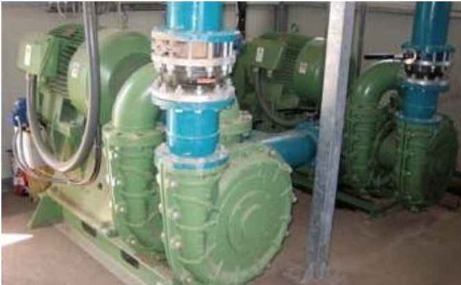
Horizontal double stage PEMO pumps for filter press
