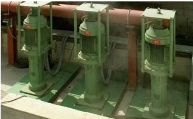
Vertical PEMO pumps for transfer of slurries
