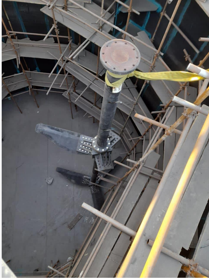
Iron Ore Tailing Agitator, 90kw, 3.7m dia
